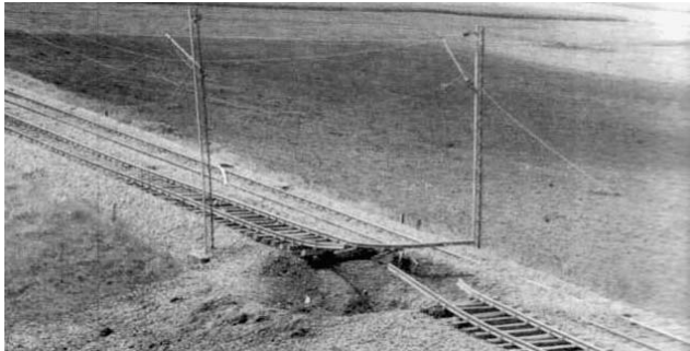
Figure 5. Broken railway tracks on the Belgrade-Skoplje railway line in the vicinity of the demolished flyover near Trupalske forest, Nis, 14 May 1999.
