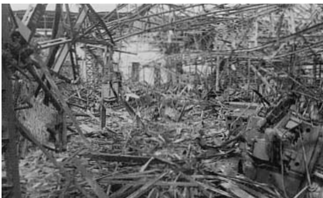
Figure 3. Inside view of demolished Zastava Trucks plant, 9 April 1999.
