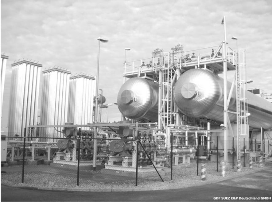
**Fig. 2.3** The interim-storage and conditioning unit near Maxdorf (Altmark). In the very front of the two 300 m<sup>3</sup> vessels, two injection pumps are installed. Four air cooled evaporators can be seen to the *left hand side*
