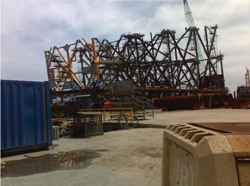
**Fig. 2.1** Jacket platform under fabrication at a yard
