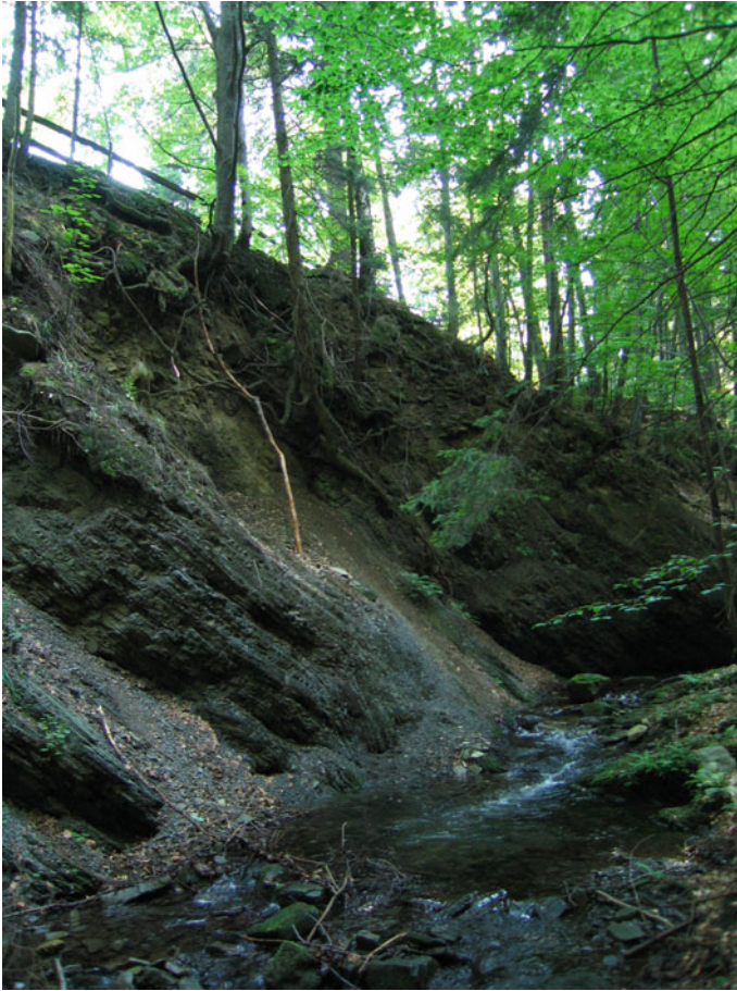
Fig. 5 A channel-reach incised 6 m into claystone bedrock downstream check dams in the Malá Ráztoka watershed (the upstream view)
