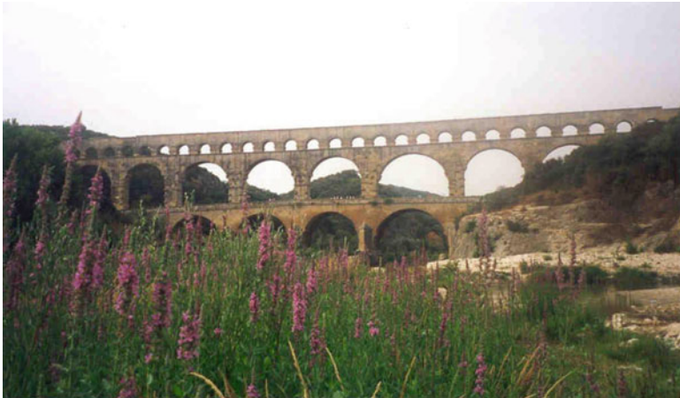
Fig. 2.5 Photo of the Pont du Gard (note people standing on the lower deck)
