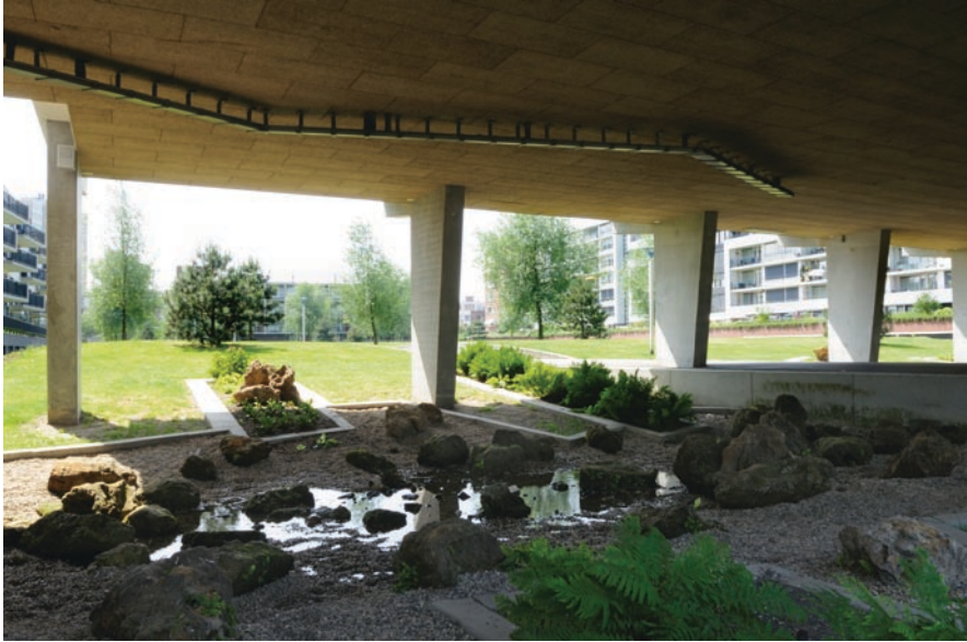
Fig. 2.1.1 Adaptation measure: a rainwater infiltration area below a building in Tilburg. A wadi ( Arabic word meaning dry riverbed that contains water only during times of heavy rain ) offers a way to deal with heavy rainfalls by buffering overflowing water and reducing the risk of flooding. In addition the wadi cools the area and offers a nice environment for plants, animals and insects (Photographer: Maartje Ansems) (see Color Plates )
