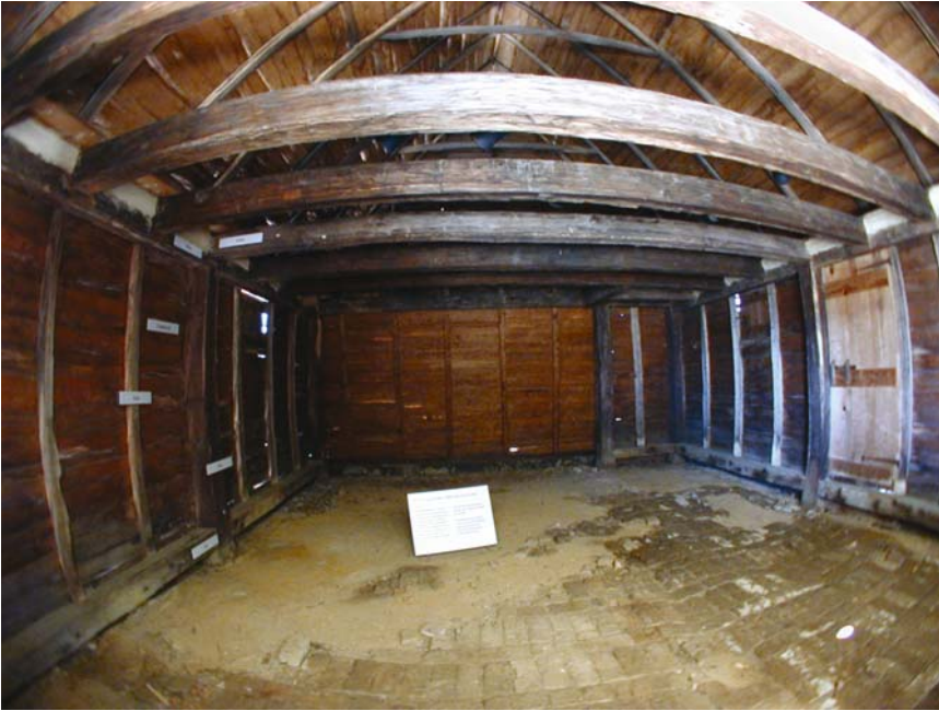
FIGURE 2.5. The reconstructed Van Sweringen kitchen with its 1690s brick floor displayed to the public. (Courtesy of Historic St. Mary's City)
