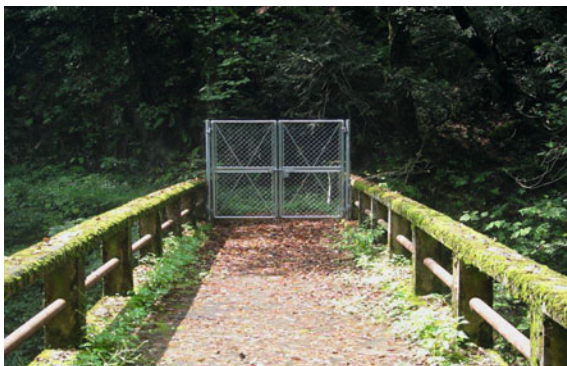
Fig. 2.4 Bridge to nowhere
