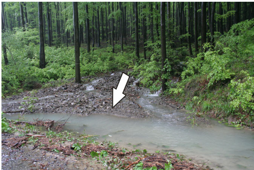
Fig. 3 A road sluice acting as a barrier to bedload transport during 5/2010 flood event due to its jamming (Lubina watershed). The arrow shows flow direction
