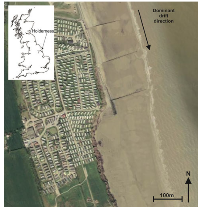
Fig. 2.1 Aerial view of the set-back downdrift of the defence works at Hornsea on the Holderness coast of Yorkshire, UK, where a 1,544 m groyne field was extended by 290 m (including a small shore parallel extension). The inset map shows the location of the Holderness coast (Photograph from Google Maps)
